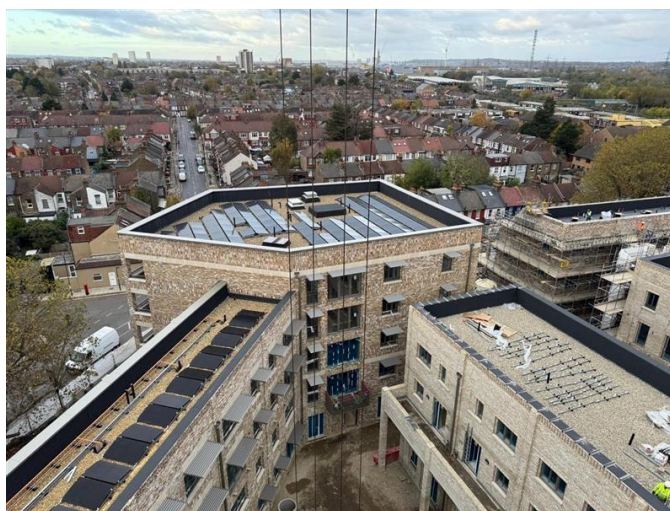
Figure 10: Image showing part of the Ashley Road development from above, with external shading, and solar PV being installed onto roof spaces.
